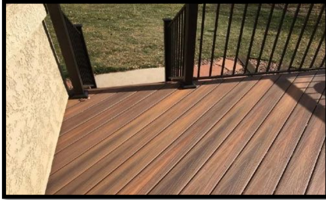
Figure 19 – Example of an artificial decking surface and metal spindles.
